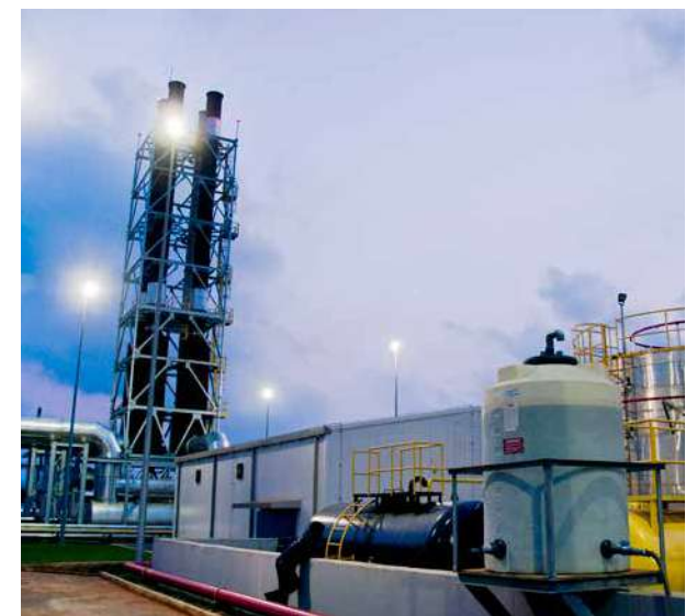
UthuruJanani Power Plant / Itl.lk
